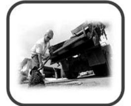
4. Compact the PHF. A compactor or roller is recommended for larger holes whilst driving back and forth with a vehicle can be used on smaller holes very effectively.
