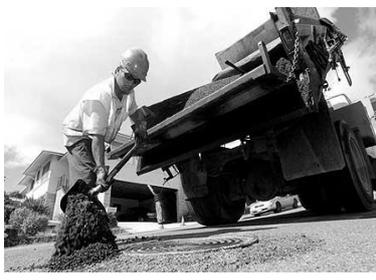
Compact pothole with a wacker packer. Deep potholes will have to be applied in layers and compacted.
