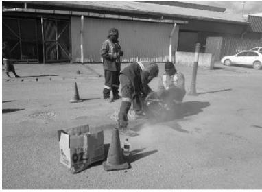
Fill the potholes 5-10mm higher than the pavement
