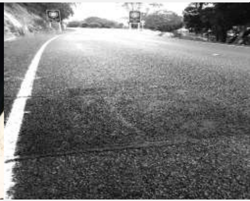
Completed Pothole Repair in Asphalt
