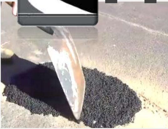
Fill pothole with premixed fill
